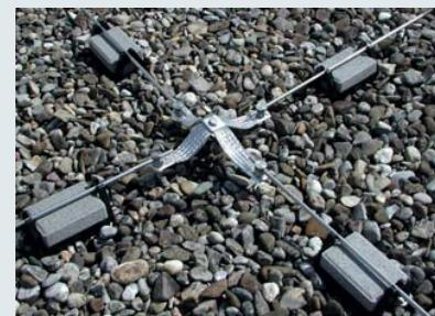
Note: At crossing points two bridging braids can be connected with a screw M10x20 mm and nut.
