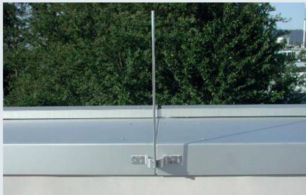
Bridging brackets for connecting and joining of metal claddings, for riveting or screwing
